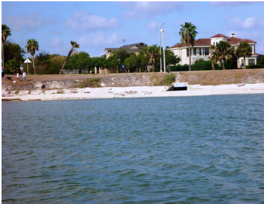
Fig. 3.15. Poenisch Park stormwater outfall (Station 21150).
