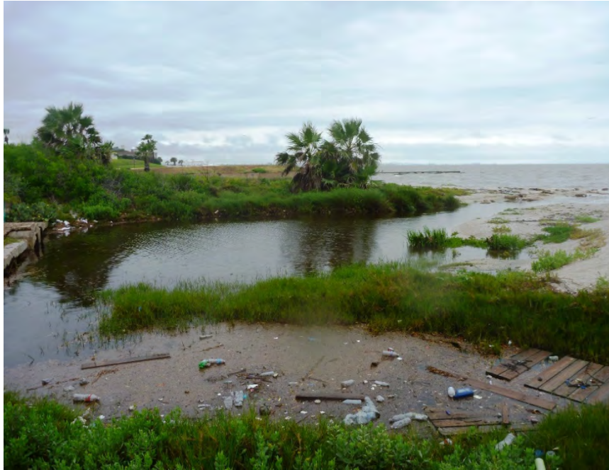
Fig. 3.14. South Shore Place stormwater outfall (Station 21149) showing large ponded area.
