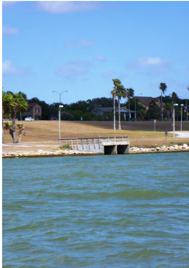
Fig. 3.8. Cole Park Louisiana stormwater outfall (Station 21143).
