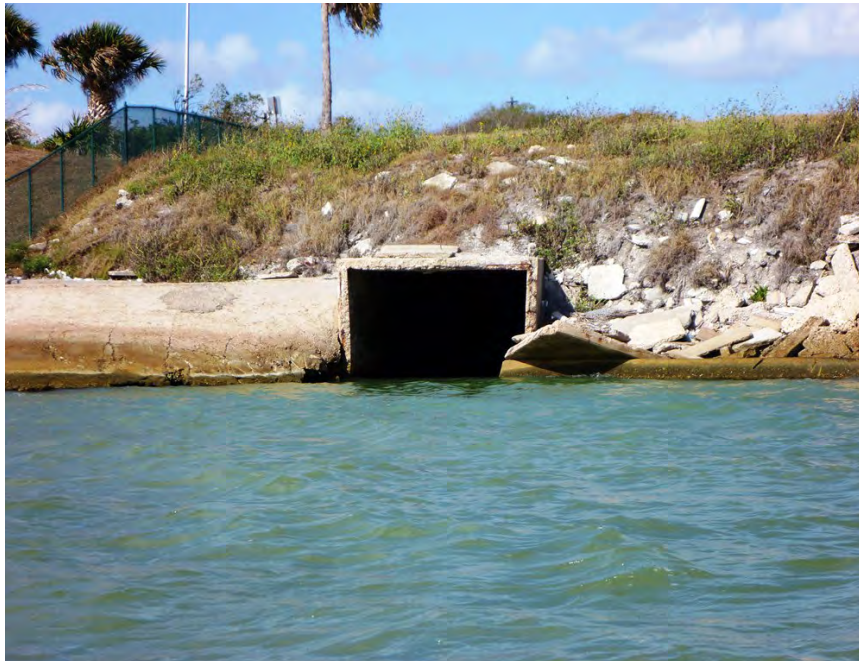
Fig. 3.11. Brawner Parkway stormwater outfall (Station 21147).
