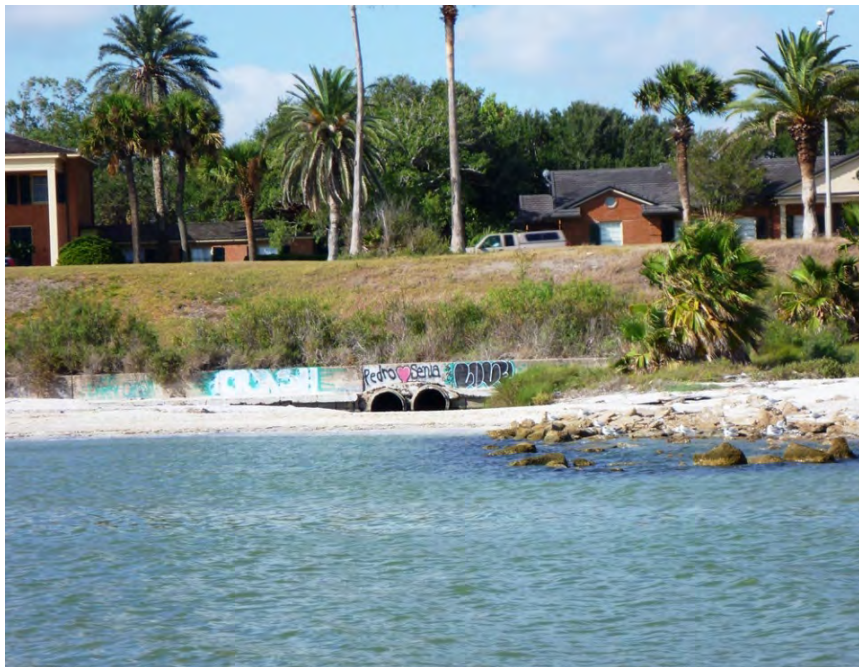
Fig. 3.13. South Shore Place stormwater outfall (Station 21149).
