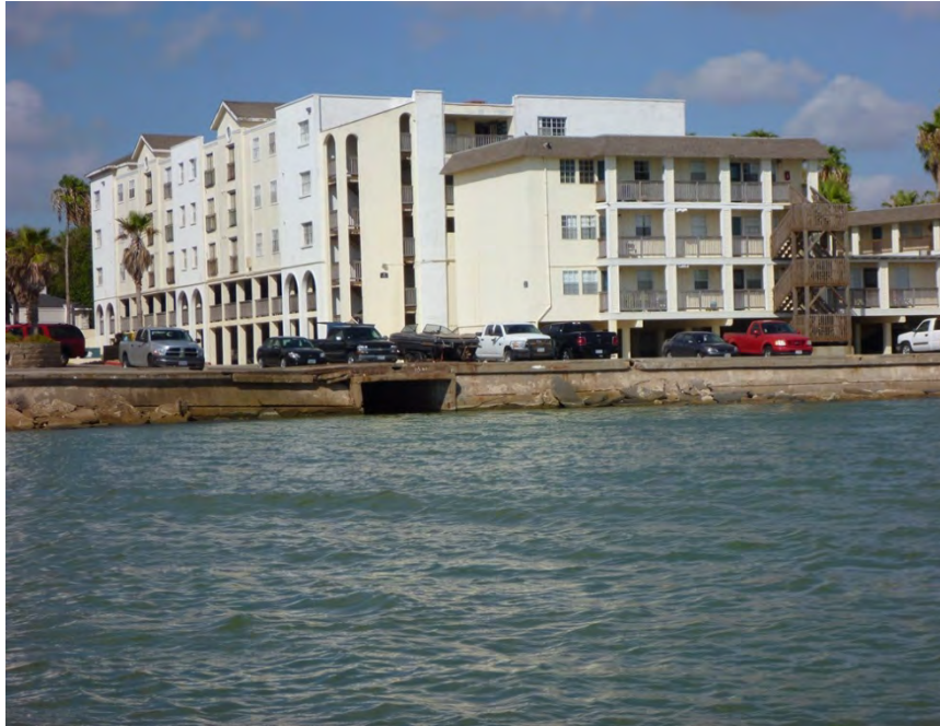
Fig. 3.12. Carmel Parkway stormwater outfall (Station 21148).
