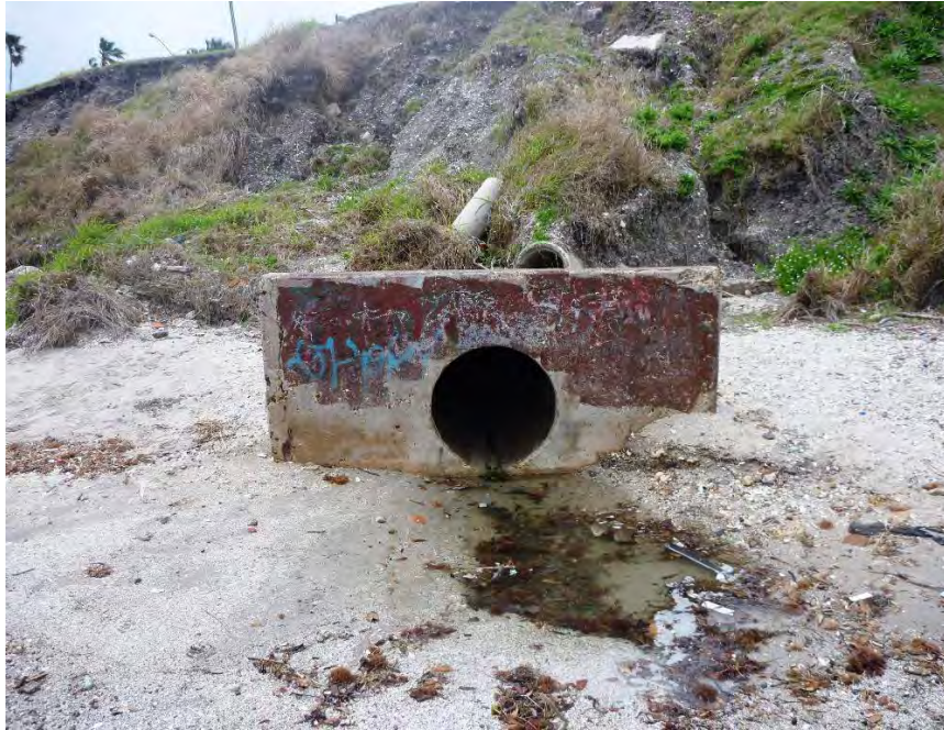
Fig. 3.10. Ropes Park stormwater outfall (Station 21146).
