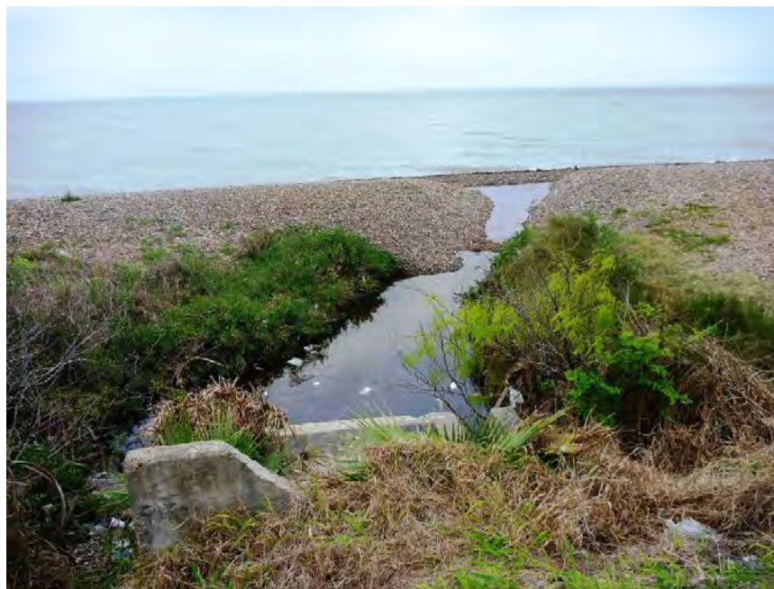
Fig. 3.9. Cole Park Oleander Point stormwater outfall (Station 21144).
