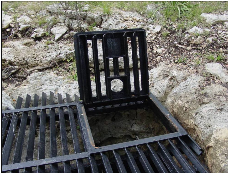
Figure 2-9. Example Cave Gate Access
