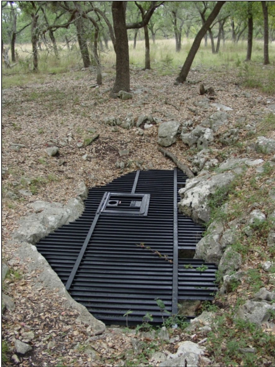
Figure 2-6. Typical Cave Gate with Secure Entrance (Mike Warton, PBS&J)
