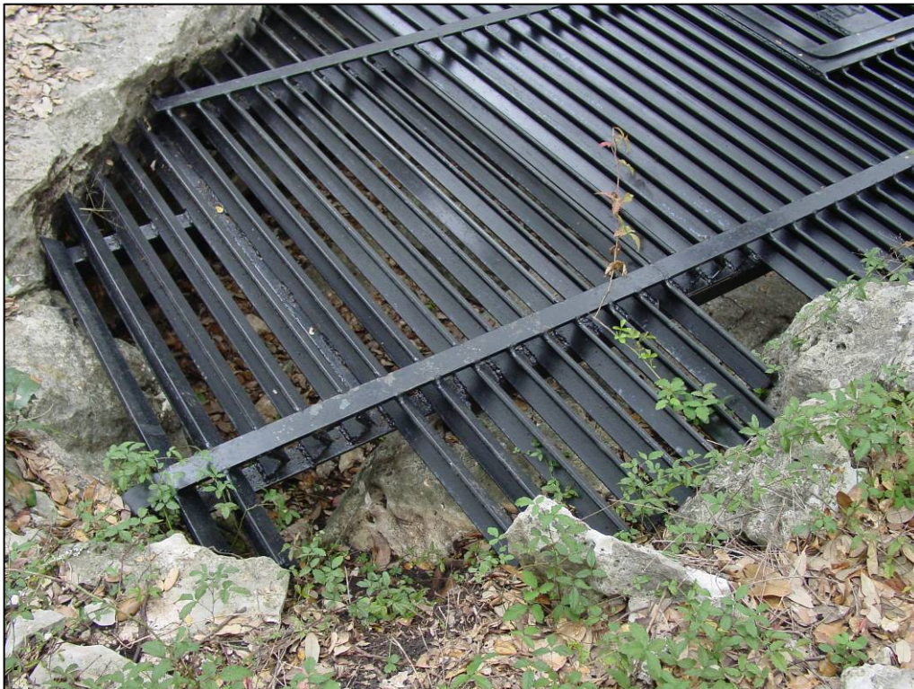
Figure 2-7. Mammal Access Portals along Edge of Gate
